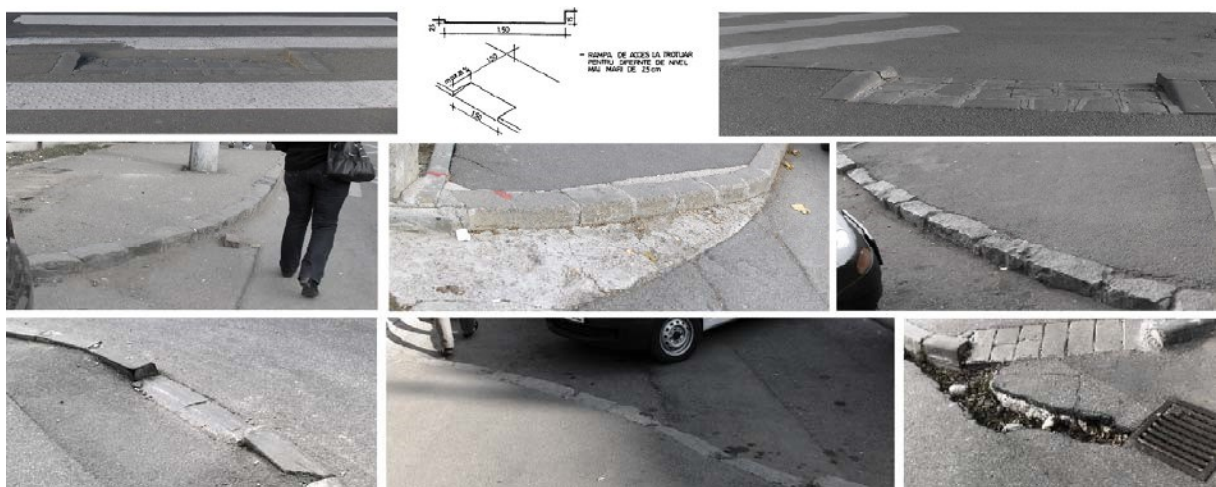
Figure 4 – Situation of access ramps on the sidewalk
